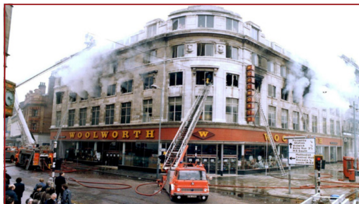
The Woolworths store fire in Manchester in 1979 involved large quantities of foam filled furniture. Ten people were killed as a result of the intense poisonous smoke produced and the fire led to the introduction of The Furniture and Furnishings (Fire Safety) Regulations 1988
